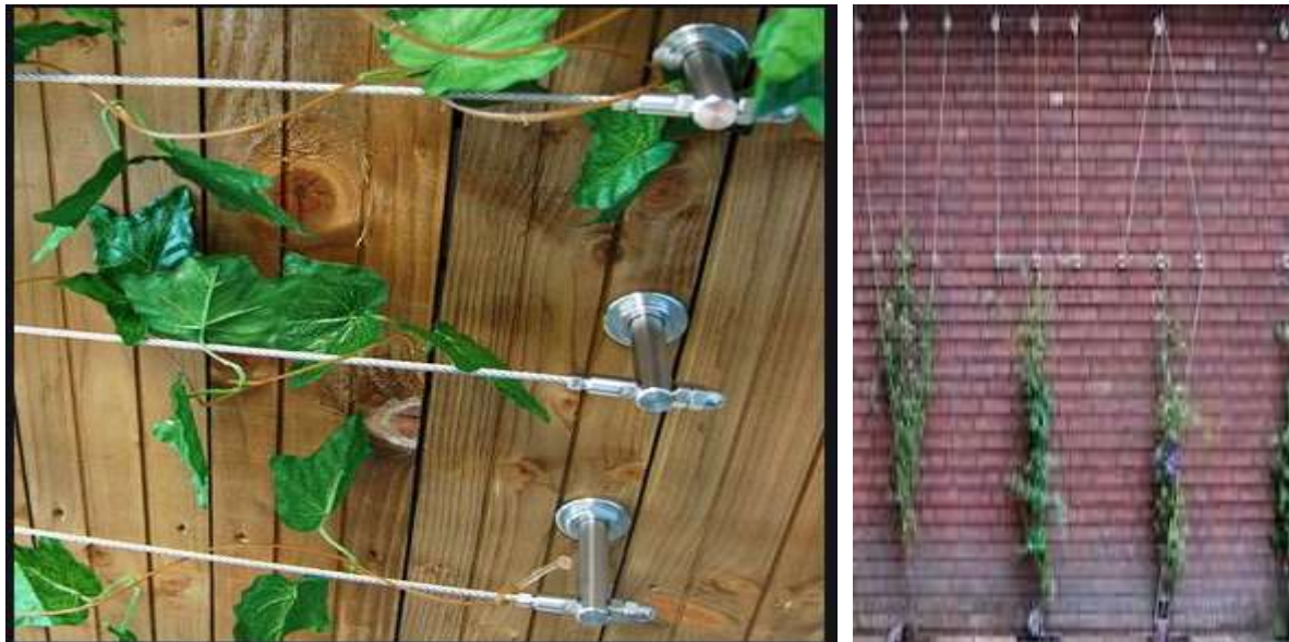
Fig.7.1 Attaching and tensioning foliage and trellis wires
